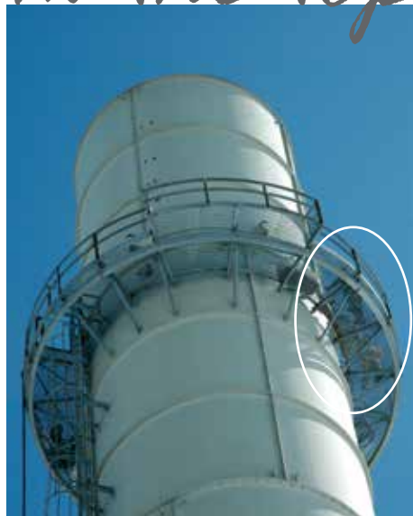
FAR LEFT: Combustion turbine stacks at an electric generating facility in Kentucky. LEFT: A ladder (on the left side of the stack) provides access to the testing platform where a test crew (circled) made the climb 150 feet to conduct a stack test. Photos by Andrea Keatley
